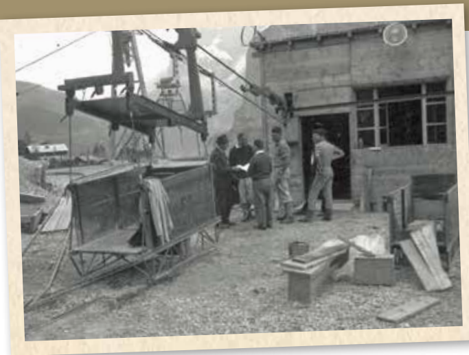
Terrifying: People too were transported to the summit by construction cableway in crates like these
