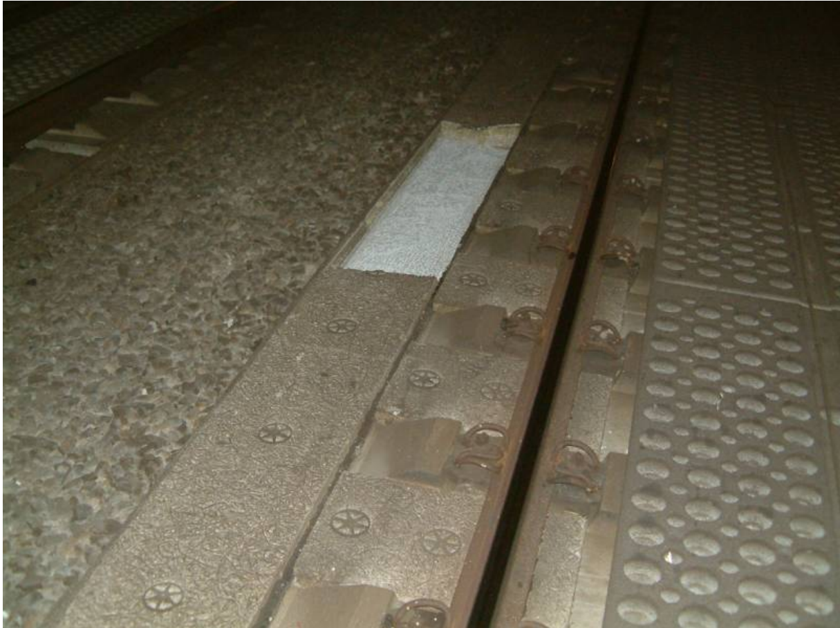
Figure 15: Damages to the protective coverings for the extinguishing water pipe
