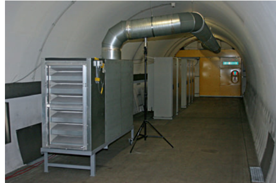
9 Filter box with measurement equipment used (flow measurements in round tube duct)
