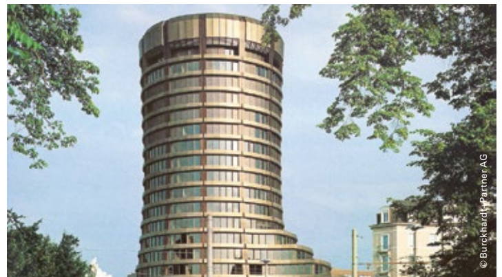
BIS tower, administrative and conference building, Basel Client: Bank for International Settlements (BIS) Project period: 1972 to 1976 Architect / lead designer: Burckhardt+Partner AG Gruner service: Structural design
