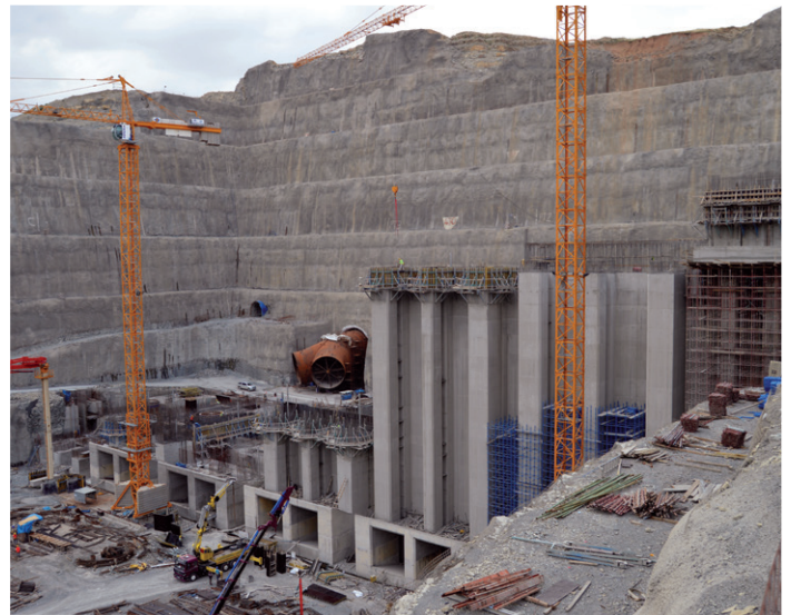
Powerhouse in construction
