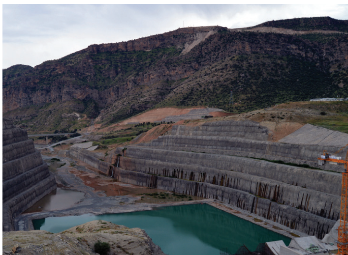
Overflow spillway flip bucket, plunge pool and tailrace channel
