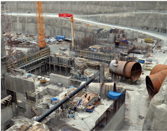
Powerhouse manifolds erection
