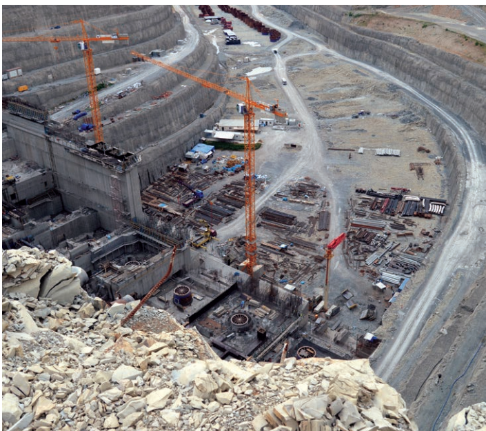
Powerhouse viewed from the upstream
