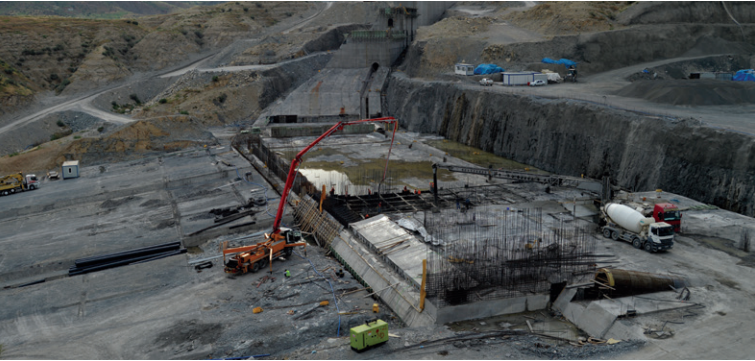
Concrete dam and spillway section
