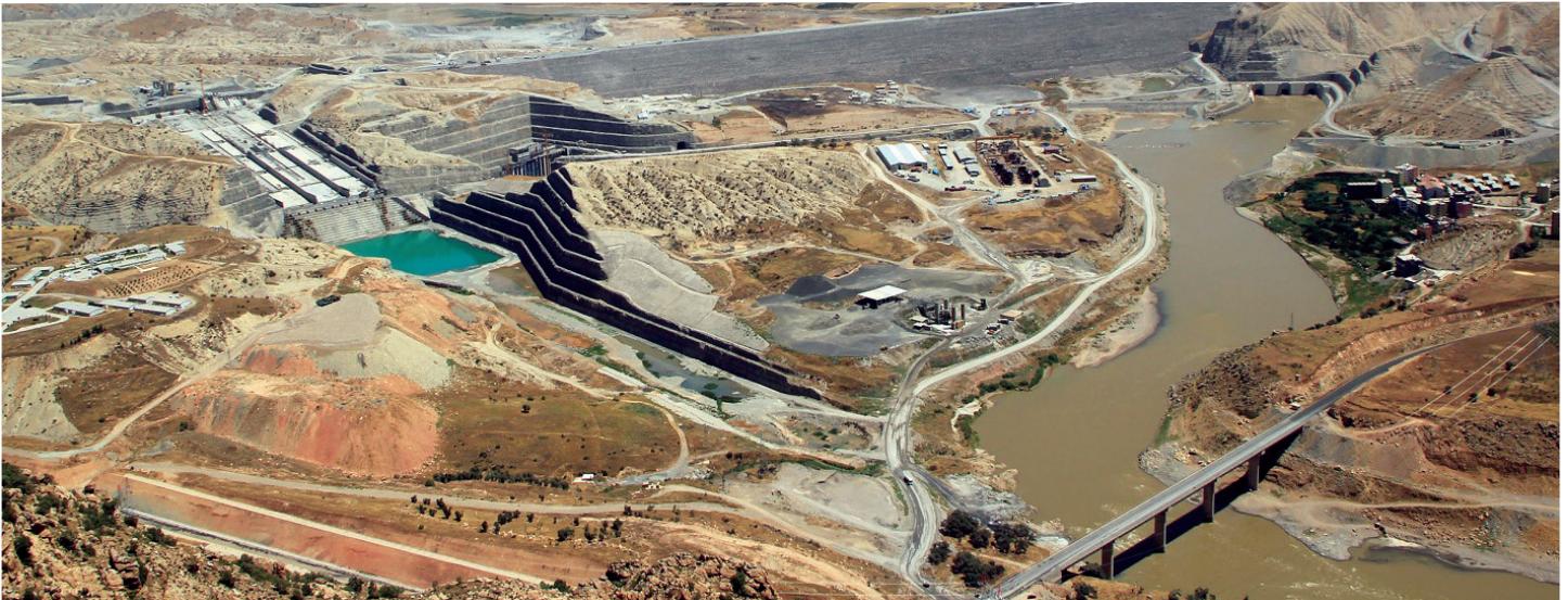
Overview of the dam site
